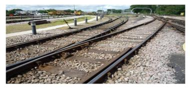
These are sections of track which do not have conductor rails.
